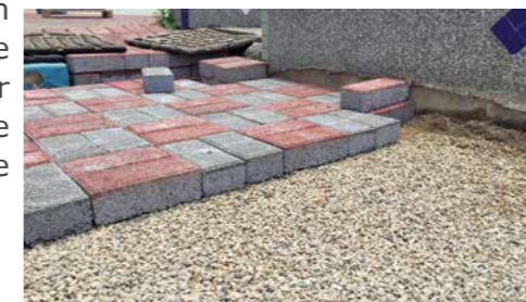
Installing a pathway with high-pressure permeable concrete block
