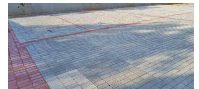
High-pressure permeable concrete block applied to outdoor parking lot.
